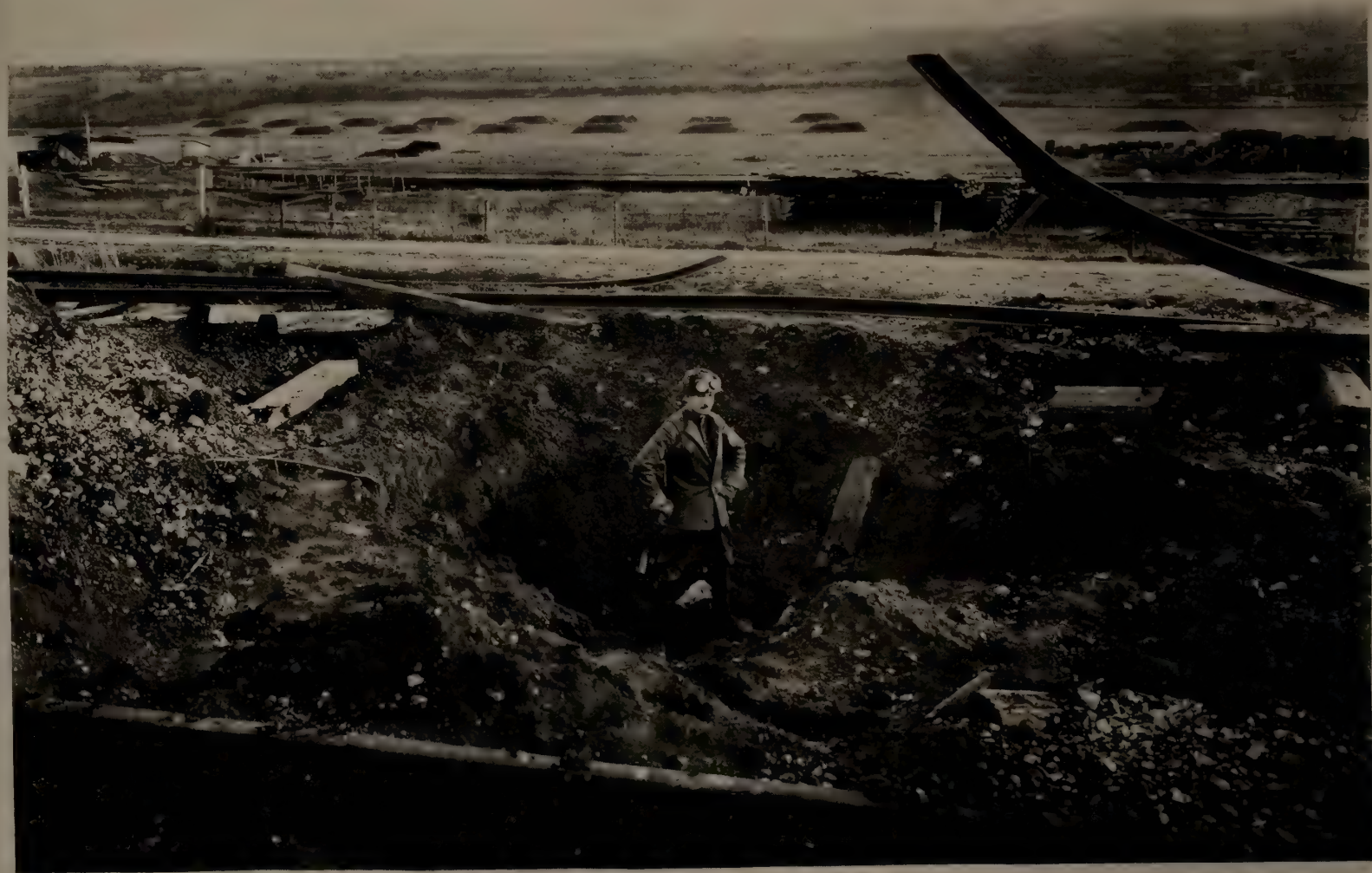
Large Shell hole in Railway bed at "Vilosnes", Notice large German Ammunition Dug-Outs in the background.
